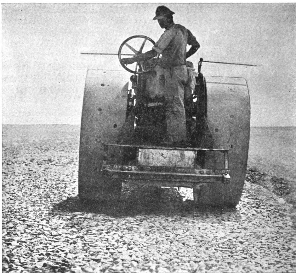
Figure 117. Compacting coarse aggregate preparatory to penetration with bituminous material.
